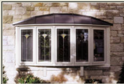
Bow Window with standing seam metal hip roof.
