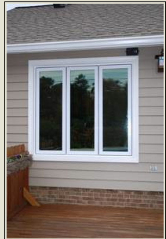
Three-section casement windows.
